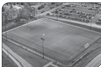
Lighted Turf Field
